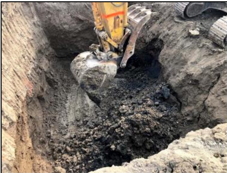
Photo of stained soils in former UST basin.
